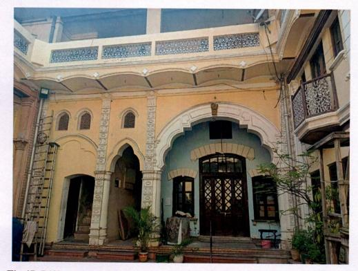
Fig.47- Different arches and Latticed screens
